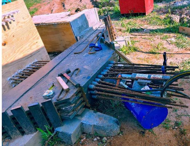
**Figure 4-9:** Pretensioning bottom strands.
