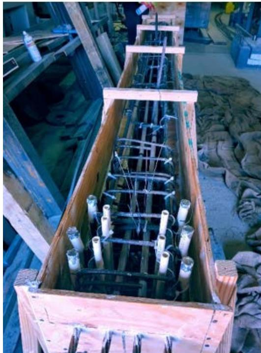
**Figure 3-15:** Reinforcement layout.
