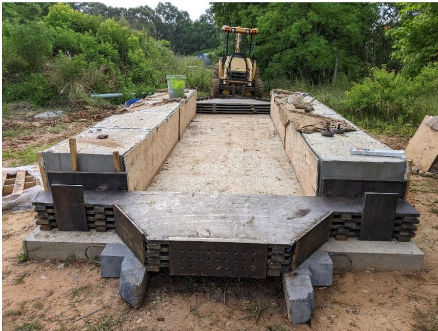
**Figure 4-4:** Prestressing bed during construction.
