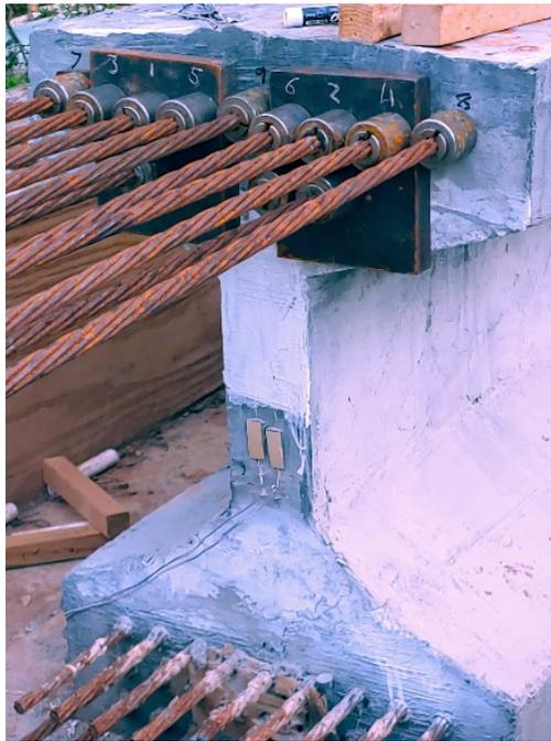
**Figure 4-12:** End of Girder A after all strands were prestressed.
