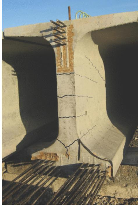
**Figure 1-1:** End zone cracks in a precast prestressed concrete beam (Okumus & Oliva, 2013)
