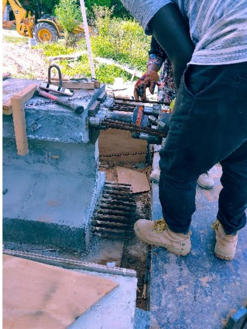
**Figure 4-11:** Post-tensioning of top flange steel strands.
