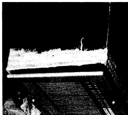
Figure 10.8 Sealant applied on the register boot.
