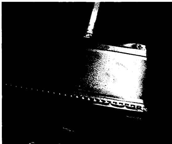
Figure 10.5 Leaks at register boot.
