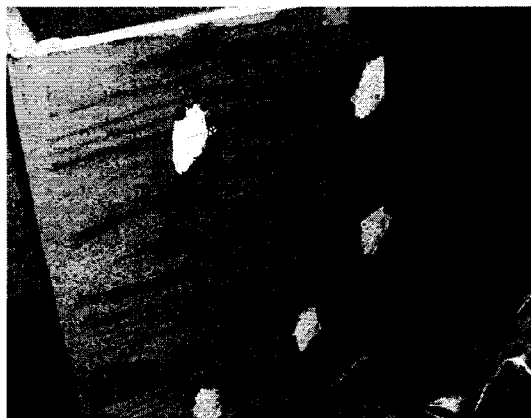
Figure 10.3 Sealant applied on drilled holes.
