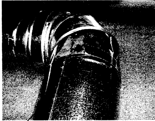
Figure 10.11 Seam of the duct system.
