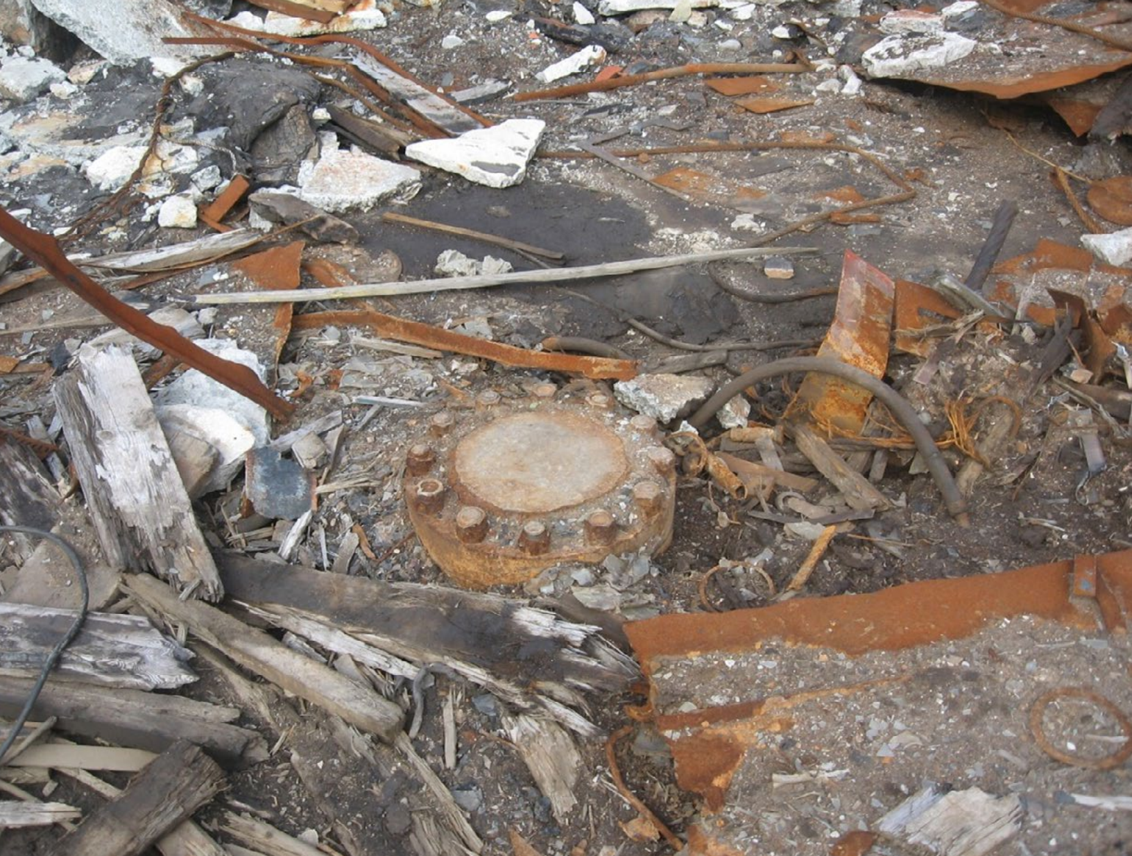
The Kola Superdeep Borehole, welded shut since project abandonment.
