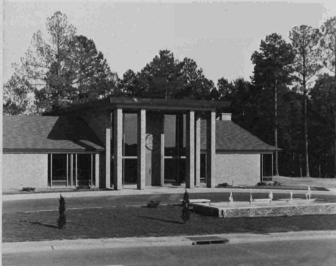
Alumni House, located just east of the new athletic complex, was financed by contributions from alumni and other friends of Tech. In front of the alumni building is the Leola Marbury memorial fountain provided by Mr. and Mrs. William Ardis Marbury, Jr., of Ruston. The fountain was presented at homecoming.
