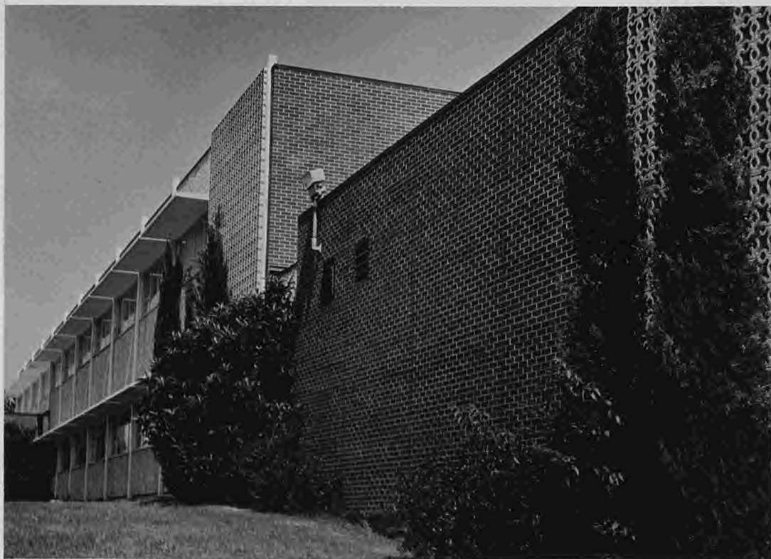
This education building, completed in 1963, was named Woodard Hall in tribute to the memory of Clifford T. Woodard, Dean of the Tech School of Education from 1956 until his death in 1966.
