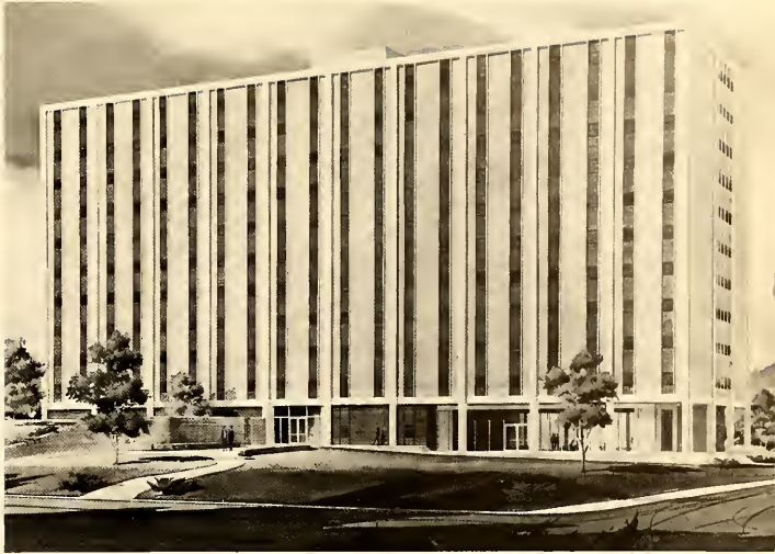
Neilson dormitory for men, under construction
