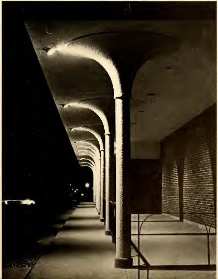
Columns of new Wilson Cafeteria
