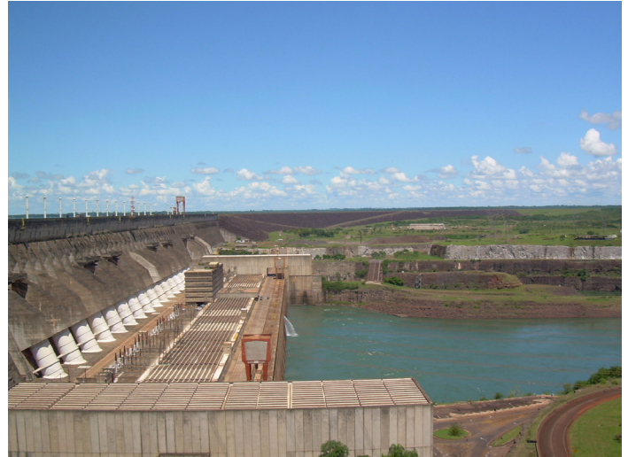
Hydroelectric plant with the generating units in white.
